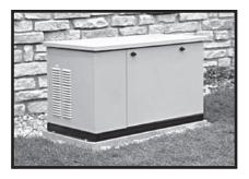
Shut OFF utility power again. The generator should start and the entire emergency load should transfer to the generator.
